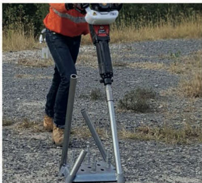
JACK HAMMER MICRO PILES
