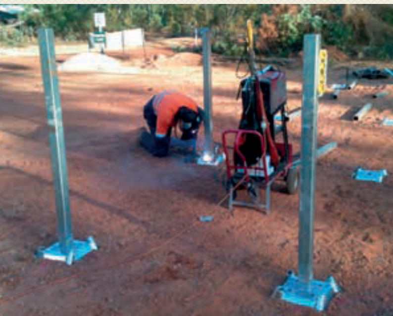
Welding directly to Surefoot
